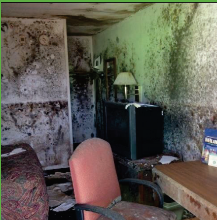
MOLD DAMAGE
